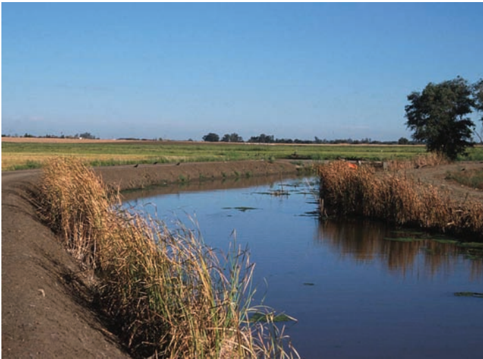
Figure 3: Timely delivery of water through over 200,000 km of irrigation canals is essential to agricultural production in the 17 western states. Aquatic weeds are also problems in concrete lined canals where submersed weeds only require a small amount of sediment to take root and grow.
